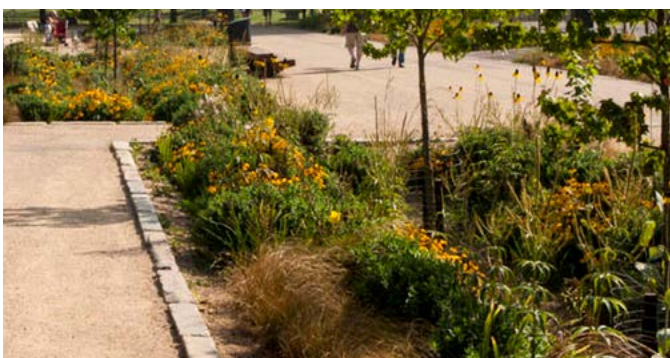
Figure 42 Sustainable Urban Drainage including rain gardens, within the design of public realm.
